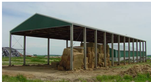
Figure 1-49. Hay storage facility with all-around access by. Post spacing on back endwall twice that on front endwall to accommodate machinery access.
