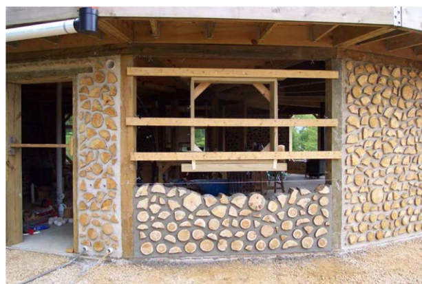
Figure 1-57. Cordwood (a.k.a. stackwood) infill walls.
