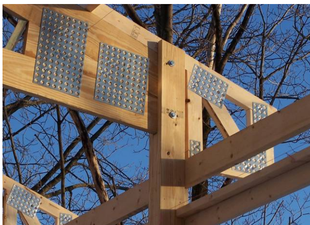
Figure 1-55. When truss is sandwiched between outer plies of a mechlaminated post, bolts are placed in double-shear for a very effective connection.
