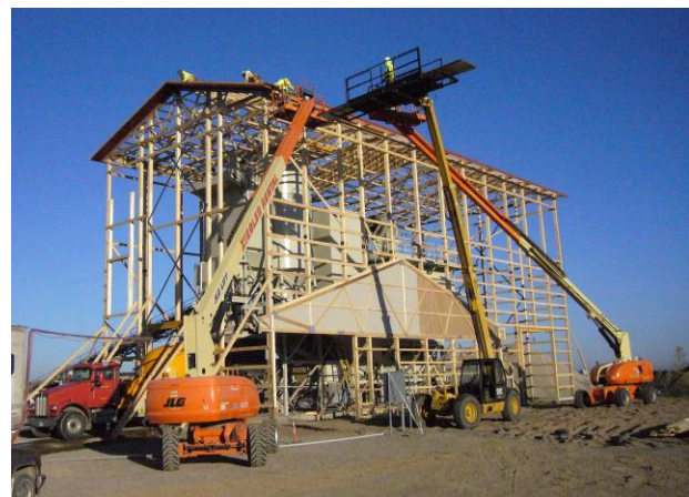
Figure 1-42. Post-frame concrete batch plant with a 45 ft ceiling height, accomplished in part by bracing wood columns back to the main structure of the concrete plant equipment.
