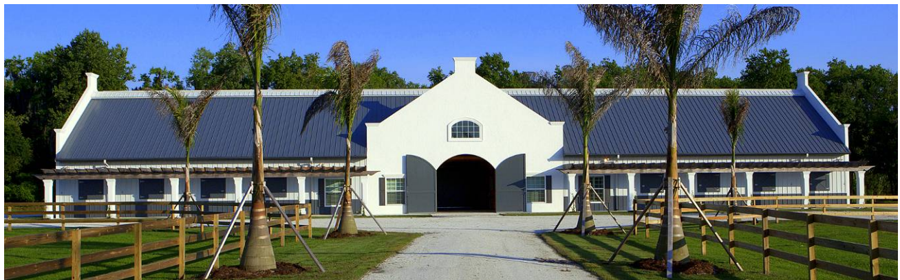
Figure 1-69. Post-frame horse barn with arcade.
