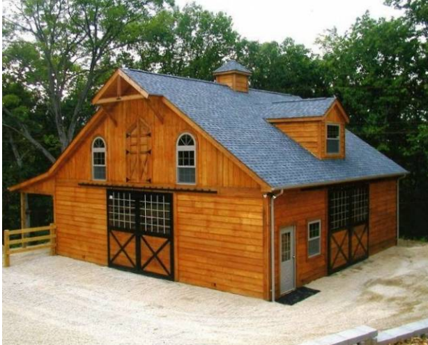
Figure 1-33. Wood-clad post-frame building constructed for horse housing.
