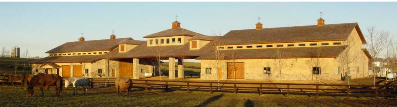
Figure 1-51. A clerestory is a common feature on many equestrian facilities.
